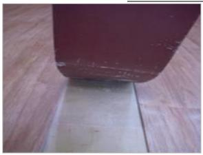
Failure – planks lifting at corners and sides.
