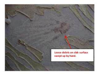
Failure – Vinyl bubbling/lifting away from slab.
